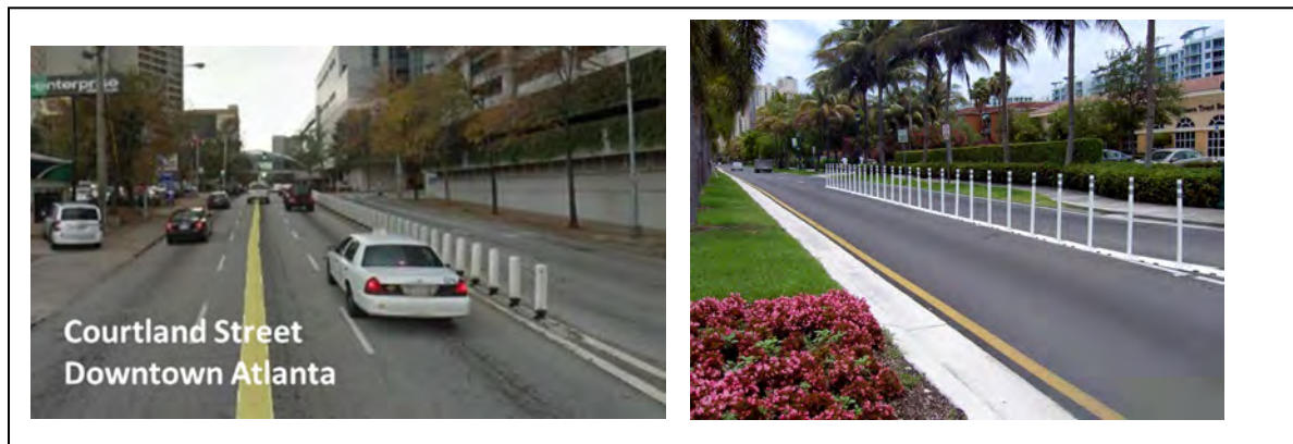
FIGURE 27. LANE RESTRICTION BARRIERS
