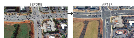
Figure 4.3. Before and After Images of Western Gwinnett Bikeway, Pleasant Hill Road and Peachtree Industrial Boulevard
